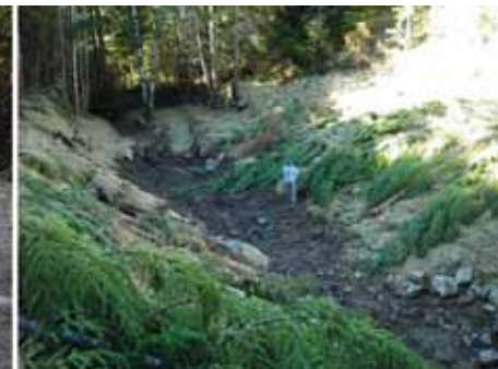
Channel after log culvert removal.
